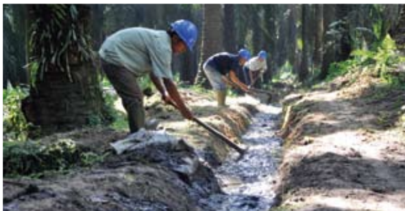
Irrigation system in plasma and core plantations
